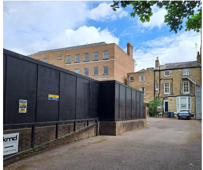
KMD rear car park off George IV Street
